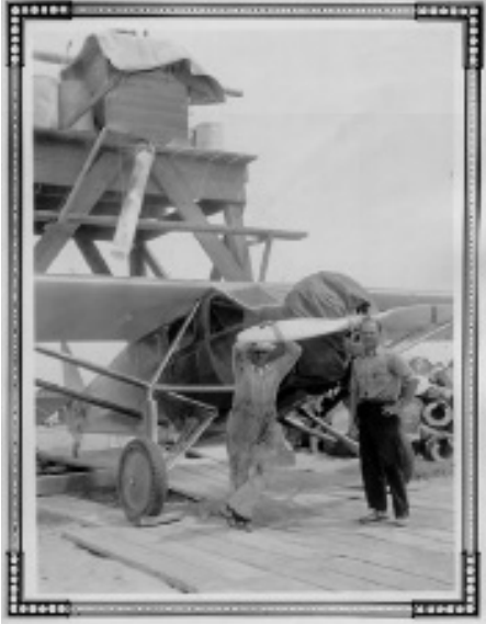
Ryan monoplane beneath a hopper and platform used for loading calcium arsenate dust to control a western hemlock looper outbreak in Pacific County, Washington, 1931. This was the first airplane dusting experiment attempted against a forest insect in western United States. (Photo 8768 by F.P. Keen, WFIWC archives). (Wickman et al. 2002, Fig. 8.)
