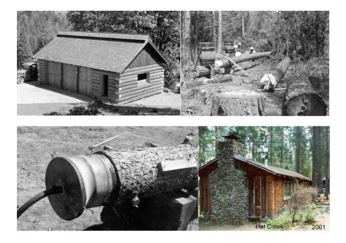
Log structure (top left) at Miami Field Base, Sierra N.F., Calif., 1939. The bark was left intact for rustic effect. To prevent insects and fungi from loosening the bark, John Patterson of the Berkeley FIL tested the effectiveness of copper sulphate & zinc chloride injected into freshly felled conifers.
